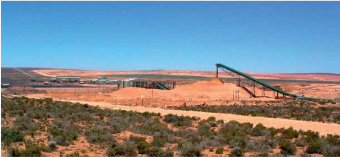
Fig. 5.1.7: Namakwa Sands operation showing primary density separation and secondary magnetic separation in the foreground and an extensive working pit in the background (Photo courtesy of Dr. D.I. Cole, Western Cape Unit, Council for Geoscience).
