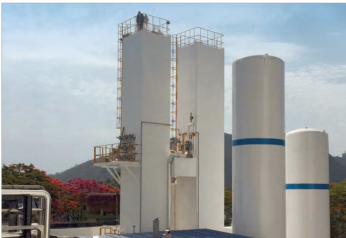
Fig. 47: The krypton and xenon purification plant in Panzhihua, Sichuan Province, of Hunan Xianggang Messer, photo: Messer Group GmbH (with kind permission).
