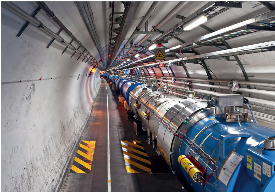
Fig. 10: View into a section of the tunnel of the LHC large hadron storage ring, the functioning of which depends on constant supercooling of the magnets by means of liquid helium, photo: Maximilien Brice, CERN.
