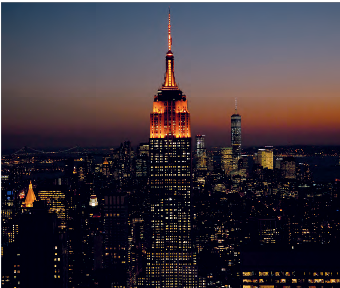
Fig. 17: In 2010, 50 of the 6379 windows of New York's Empire State Building were removed every night, one after the other; the glass interstices were coated with a metal film, then filled with a gas mixture consisting of air, argon, and krypton, and subsequently reinstalled. This reduced heat loss through the windows by 75%, photo: UN Women/Ryan Brown.
