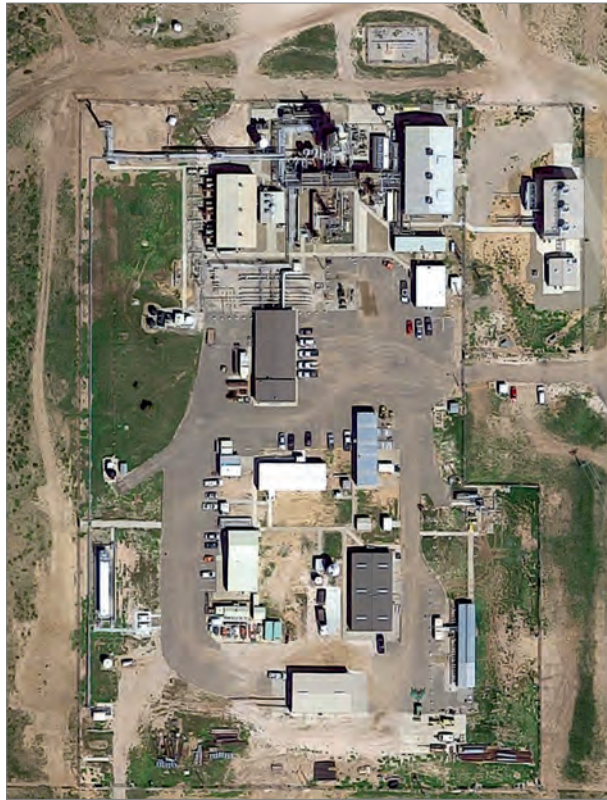
Fig. 56: The Crude Helium Enrichment Unit (CHEU) on the Cliffside storage facility north-west of Amarillo, Texas, USA, seen from space, photo: Google Earth.
